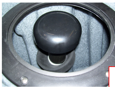
Float Shutoff Assembly
