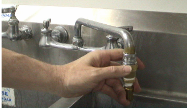
Connect the Auto-Fill Water Supply Hose to a faucet and turn on the water
